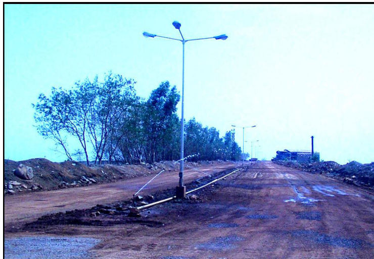
WATER SPRINKLING ON HAUL ROAD
